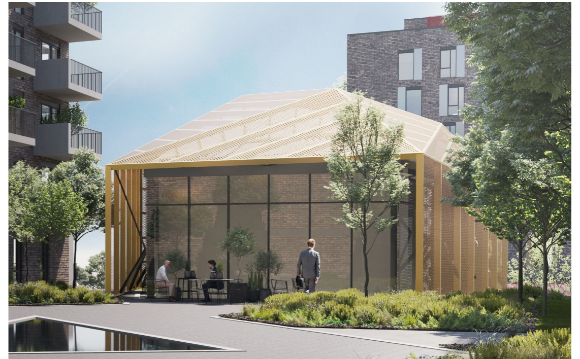
Reference images for independent structure with expressive folding perforated metal cladding structure finished with distinctive colour treatment
