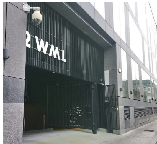
▲ Reference of a contemporary powdercoated steel carpark entrance gate with integrated clear wayfinding signage
