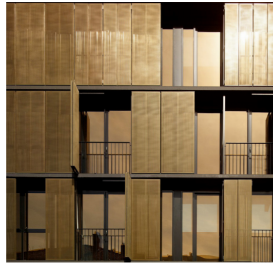
▲ Reference of anodized cladding to form a secondary screen to recessed balconies for material animation
